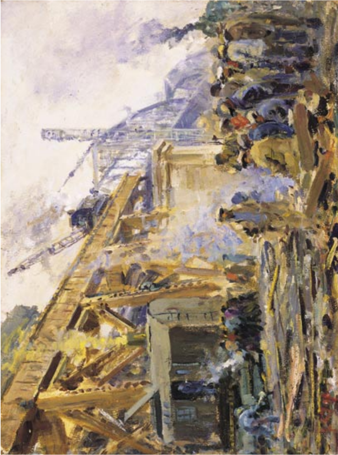
Louis C. Vogt, C&O Railroad Bridge Construction , ca. 1929, Museum Purchase. Purchase: Bequest of Mr. and Mrs. Walter J. Wichgar, 2002.129
